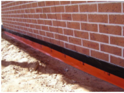
photo 1 installed against slab edge
