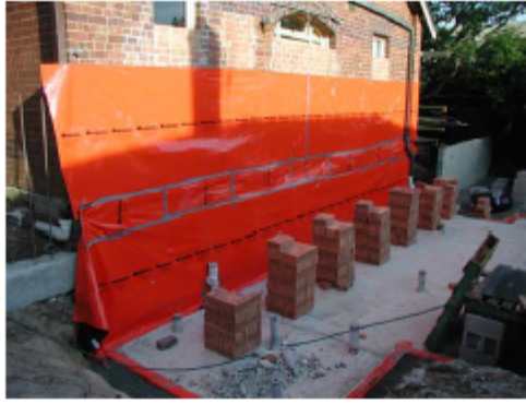
photo 1 showing existing structure with Kordon TB secured as per sketch
