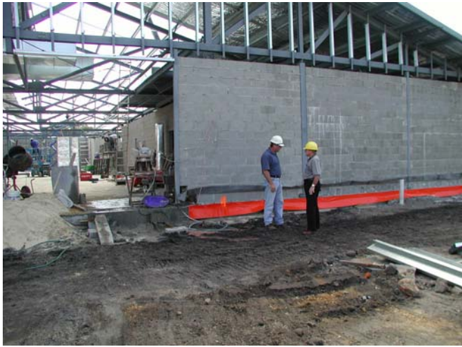
Photo 1 Kordon TB -commercial building
